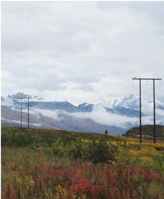
New T-Line, Thompson Pass, Dale Orvedahl, CVEA
