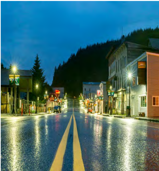
Beauty of Underground Electricity, David Little, CEC
