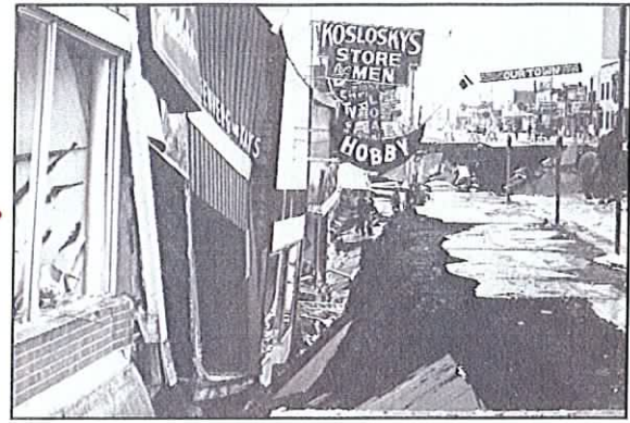
Earthquake damage in Anchorage.
