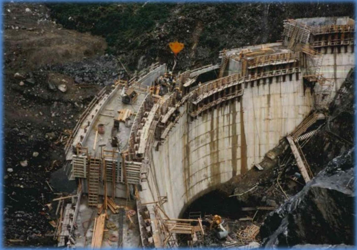
Swan Lake Dam Construction 1983
