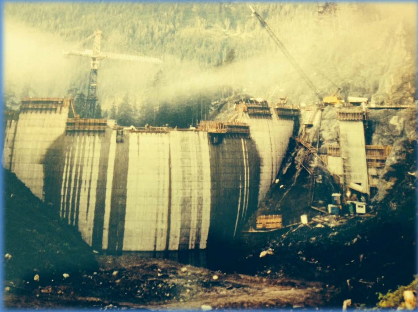
Swan Lake Dam Construction 1983
